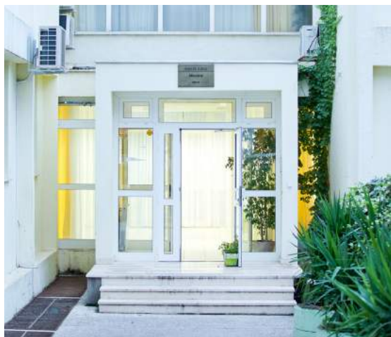
The exterior of the apartment building the Young Living Foundation plans on purchasing for its partner organization, the Maestral Orphanage
